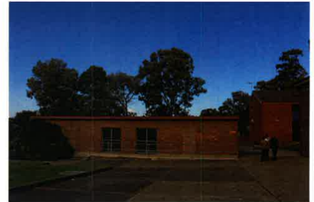
View of proposed demolition of existing toilet blocks.
