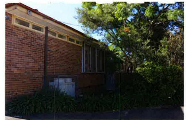
View of the back of the administration building. Extension and refurbishment works are proposed for this building. Extension of admin will be located here.
